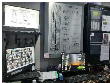
Graphic Annunciator Fire Alarm System
